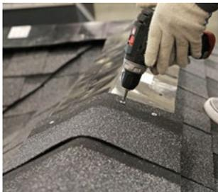
Cut hip & ridge shingles to the width of the ridge vent and fix them through the vent directly to the base with galvanized self-tapping screws with washers using **4 pieces** per element.
