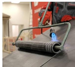
Then torch the remaining part of the membrane. Direct the flame to the place where the membrane touches the base, uniformly heating the material across the entire width.
