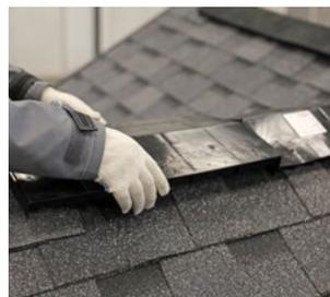
Fix the ridge vents to the base with galvanized self-tapping screws of **60 mm** length.
