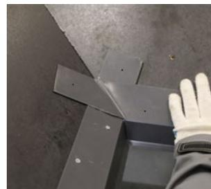
Form the outer and inner corners by joining the planks together.
