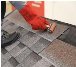
Torching of the following rows of shingles is performed end-to-end to the previously installed ones. Press the lower part of the shingle, turn up the upper part with the spatula and torch. Then, press it with the roller.
