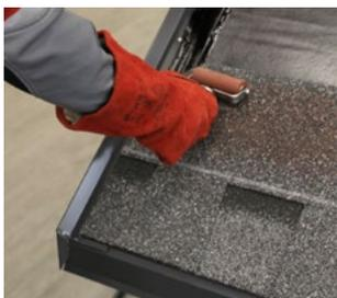
After torching, press the shingle with the roller. Do not cut the part of the shingle, which comes to the opposite slope.
