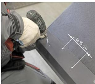
Eave and fronton overhangs are reinforced with metal planks. Fix the planks every **12-15 cm** in staggered order. The planks should overlap on each other by **3-5 cm**. Depending on the base type, the planks are fixed with galvanized self-tapping screws or dowel-nails.
