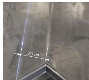
At first, mark a line with the chalk reel on a steeper slope at the distance of **20 cm** from the valley center. For convenience, cut the shingles along this line before installation. Shingles corners coming on the fronton plank are clipped by **2-3 cm** to keep water flowing downhill.
