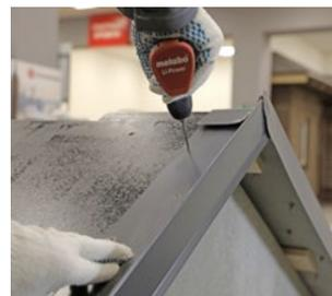
Fix the fronton planks with an overlap on the eave planks. Note: if the roof slope is from **5°** to **12°**, the fronton planks are installed before torching the underlay membrane to the decking.
