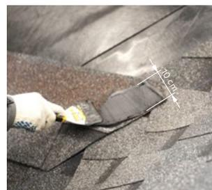
Coat the shingles overlap area with mastic TECHNOMICOL FIXER to the width of **10 cm** before torching. The thickness of the layer should not exceed **1 mm**. Do not torch the coated area of shingles overlap.
