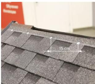
When getting to the ridge, do not torch the last row, but cut it in place and fasten with a span of **15 cm** using self-tapping screws with washers.
