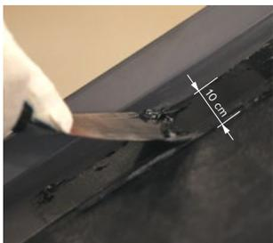
Before torching, coat the area of shingles overlap on the fronton plank with mastic TECHNOMICOL FIXER to the width of **10 cm**. The thickness of the layer should not exceed **1 mm**. Do not torch the coated area as the mastic itself will provide the required adhesion with the roofing shingles.
