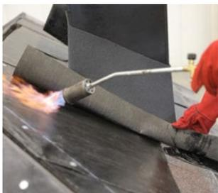
Torch the cutouts of the valley roll material overlapping the underlay membrane.
