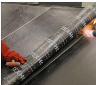
Before torching, roll one half of the membrane to the valley center and then torch it with gradual unrolling of the material along the slope. The torch should be oriented directly to the place where the membrane touches the base. Press the material with the silicone roller at the center of the valley.
