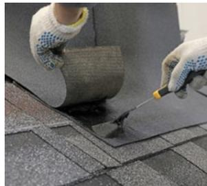
Coat all overlaps of valley roll material with mastic TECHNOMICOL FIXER. Do the same for joints between the valley roll material and the roofing shingles.
