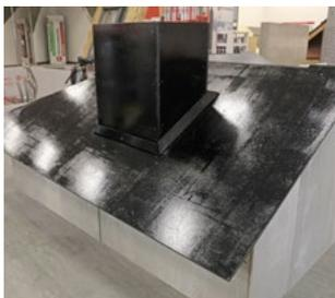
After priming the surface, leave it to dry. Drying time depends on weather conditions during the works and usually does not exceed **12 hours** at a temperature of **20 °C**.
