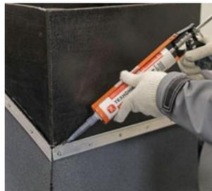
The junctions of the valley roll material with the chimney should be covered with metal flashings and then sealed.
