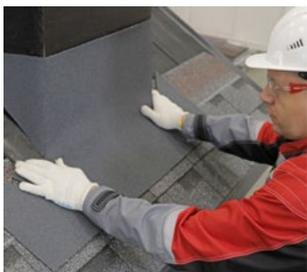
To seal the chimneys and vent pipes, prepare the cutout of the valley roll material by TECHNOMICOL, coat it with mastic FIXER and attach, observing the cascading.
