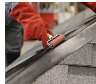
Then torch hip & ridge shingles to that strip from the bottom upwards, observing the cascading. Remember to direct the flame of the torch to the underlay membrane only. The next shingle should overlap the previous one for **3-5 cm**.
