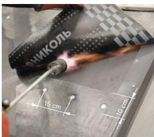
Horizontal overlaps with a width of **10 cm** are also additionally fixed with a span of **15 cm**.
