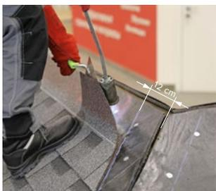
Cut the shingles adjacent to the hip at a distance of **12 cm** to each side of the hip axis and perform the regular torch-on installation.
