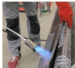
Torch the underlay membrane on the roof slopes from the bottom upwards. At first, torch the material in the eave zone.
