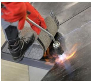
Then align the first shingle to the membrane leaving **1-2 cm** to the edge of the fronton plank. Press one side of the shingle and torch the other side.
