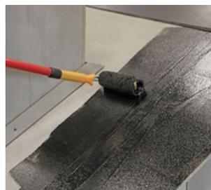
In order to provide reliable adhesion of the underlay membrane to the surface, apply a thin layer of BITUMEN PRIME COATING by TECHNOCOL with a fur roller.
