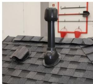
For installation of penetration elements on the roof, it is necessary to provide through holes in advance during the construction of the decking.
